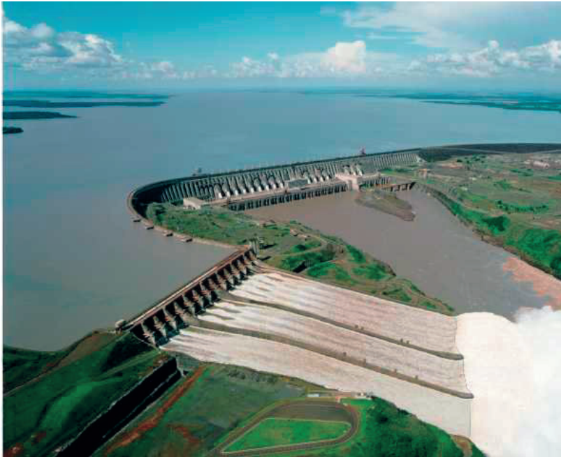
Dam at Itaipú- Iguazú (Brazil)
